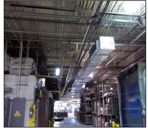
New duct installed with minimal impact on plant production
