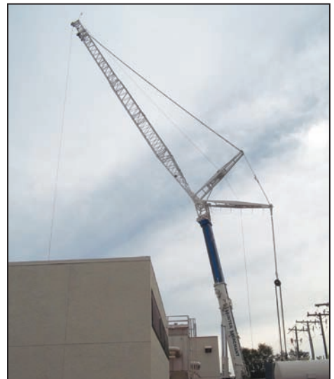
800 Ton Crane with 500 foot boom
